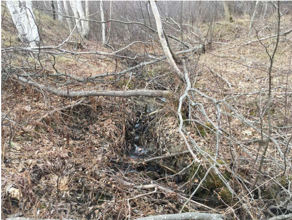
PICTURE 5: VP 1 Inlet (looking northwest up stream)
